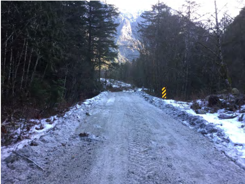
Approach from Right Bank when facing downstream
