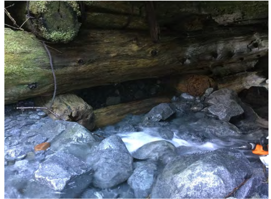
Left Bank Abutment when facing downstream
