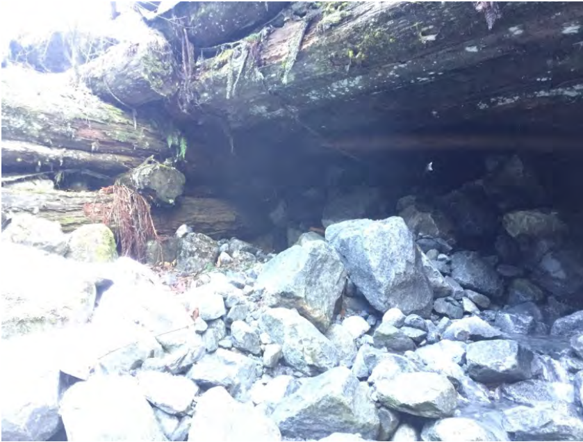
Right Bank Abutment when facing downstream
