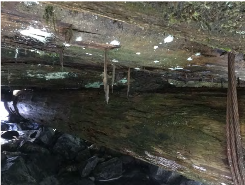
Non functional needle beam
